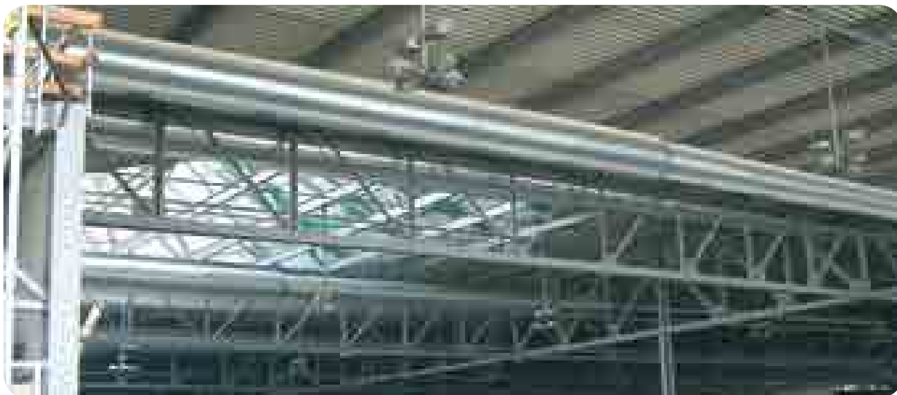
MILAN POLO EXHIBITION CENTRE, RHO-PERO. CIRCULAR Ø 630 TO 1500 MM VENTILATION DUCTS AL CLAD SYSTEM WITH K- FLEX ST ELASTOMERIC SHEET
