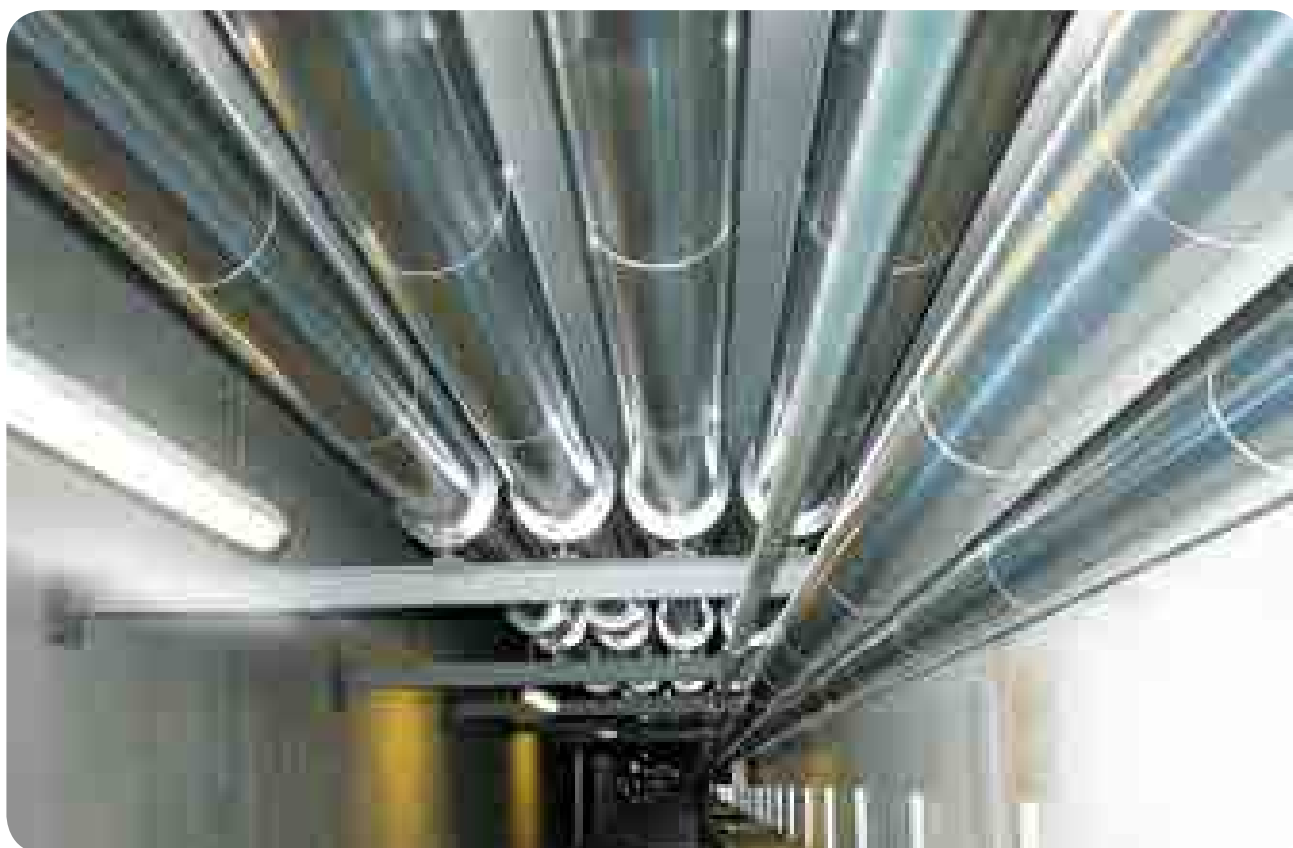
MONZA RACING TRACK. PIPES AL CLAD SYSTEM WITH K-FLEX ST ELASTOMERIC SHEET
