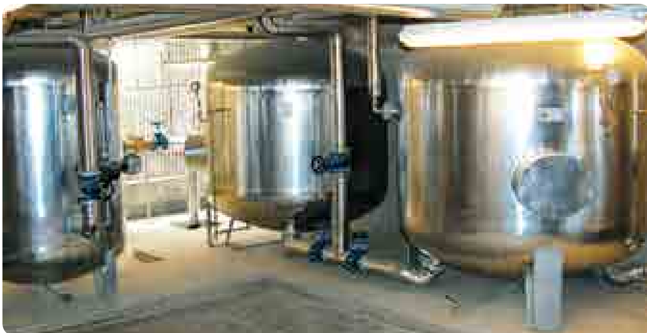
PIRELLI HEADQUARTERS, MILANO. TANKS AL CLAD SYSTEM WITH K- FLEX ST ELASTOMERIC SHEET
