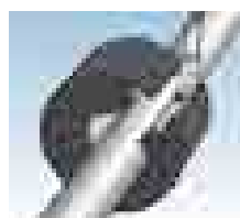
2 - Spread K-FLEX adhesive onto the half-collars.
